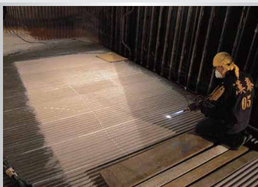
爐管施工 (Furnace Tube Construction)
