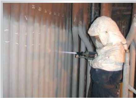
鍋爐水管牆熔射 (Water Wall Tube HVOF Spraying)
